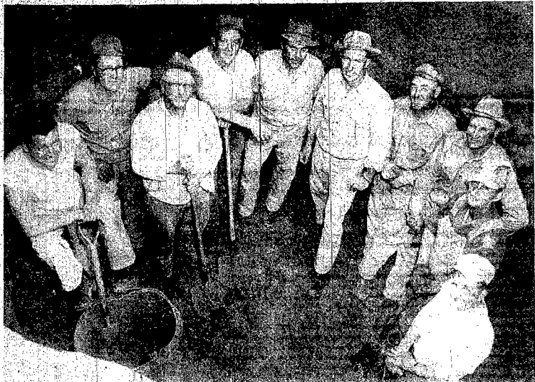
A modern public restroom will be open at Wayne county fairgrounds this summer, built mostly by volunteer labor. Shown above is part of the crew of men who excavated for the water storage tank last week at the rear of the 4-H building. Standing from left to right at the bottom of the hole are: Gene Fredrickson, Al Topp, Al Bahe, Ray Roberts, Jr., Herb Perry, Marvin Dunklau, Felix Dorsey, Marty Willers, Henry Doting and Ken Splittgerber. John Mohr had been helping but was absent when the photo was taken. Topp is from Pilger and Roberts is from Wakefield. The rest of the men are from Wayne.
